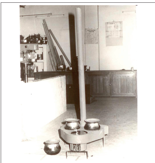
VIEW OF A WOOD BURNING STOVE DEVELOPED AT CPRI UNDER NATIONAL IMPROVED CHULA MISSION 1983
