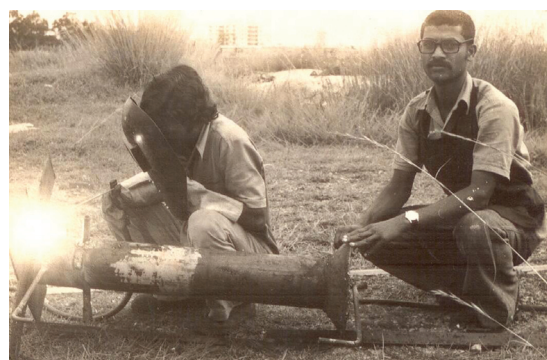
STEAM OPERATED PISTONLESS PUMP CONSTRUCTION 1981
