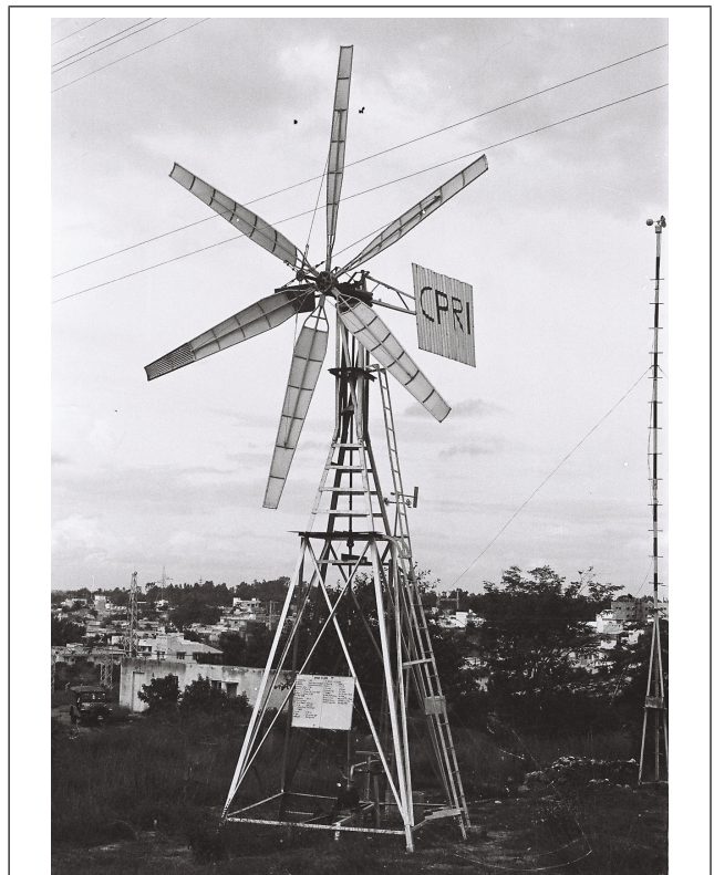
WATER PUMPING WINDMILL 1985
