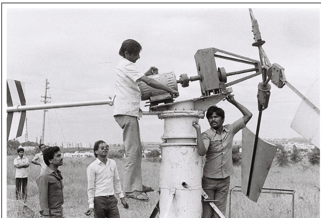
WIND ELECTRIC GENERATOR 1984
