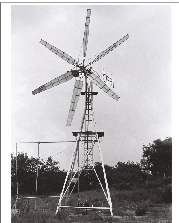
WATER PUMPING WINDMILL 1985
