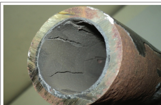
HEAVY OXIDE SCALE GROWTH LEADING TO OVERHEATING AND CONSEQUENT FAILURE
