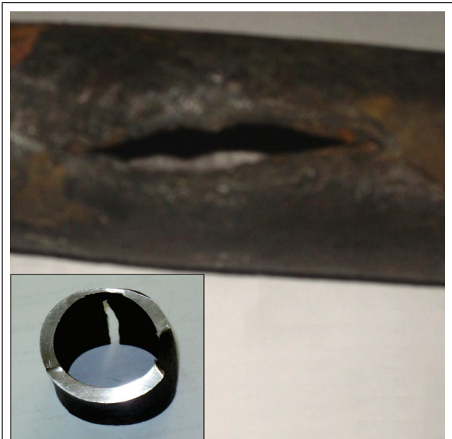
FAILURE INVESTIGATION OF THINNING IN BOILER TUBE
