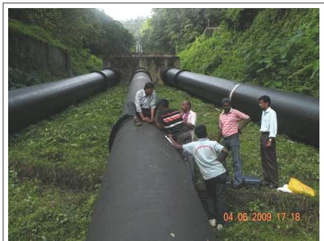
ULTRASONIC TEST ON THE PENSTOCK PIPES
