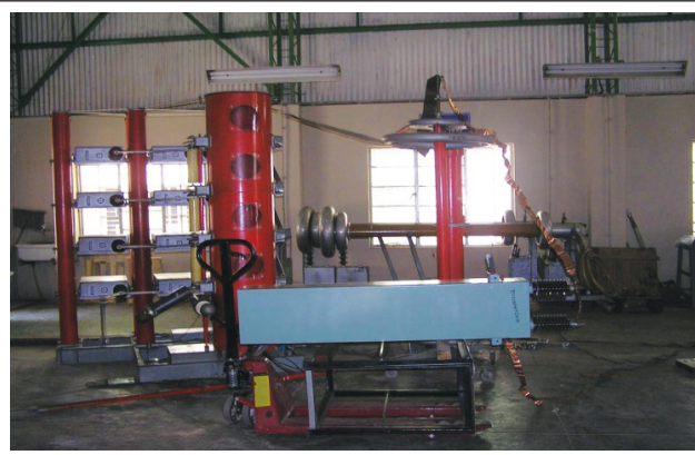
FIG. 15 A VIEW OF LIGHTNING IMPULSE VOLTAGE TEST BETWEEN CAPACITOR TERMINALS AND CONTAINER
