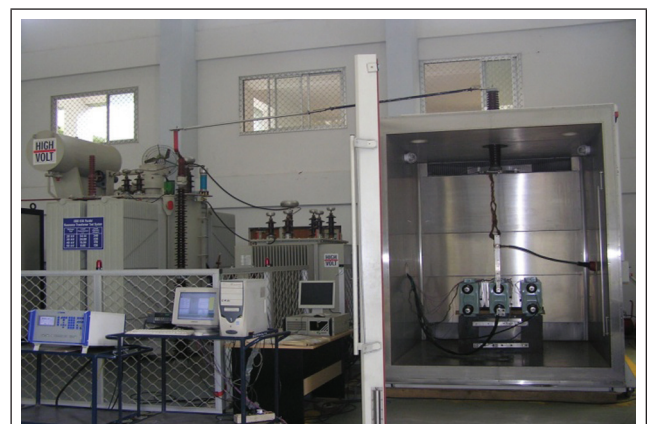
FIG. 14 ARRANGEMENT FOR THERMAL STABILITY TEST ON 1118 kVAr, 12 kV SHUNT CAPACITOR
