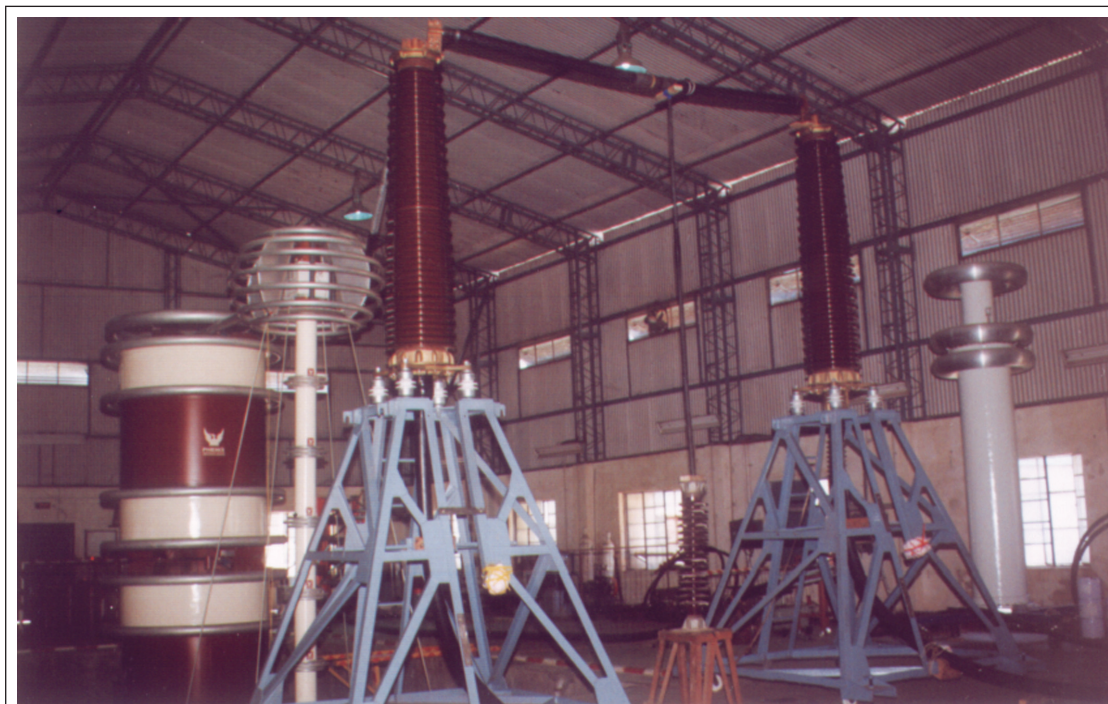
FIG. 24 TEST SET UP FOR 220 kV CABLE SYSTEM
