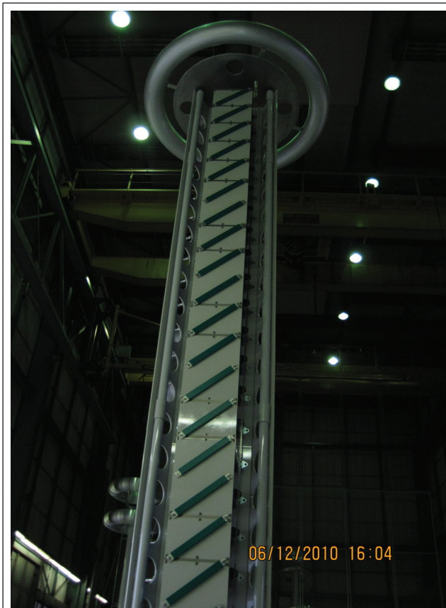
FIG. 25 A VIEW OF 2400 kV, 240 kJ, IMPULSE GENERATOR
