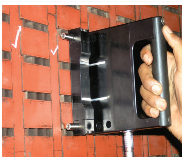
A VIEW OF WEDGE MAPPING TEST ON GENERATOR IN PROGRESS
