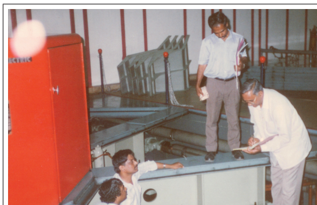
GENERATOR INSPECTION OF IDUKKI UNIT 1
