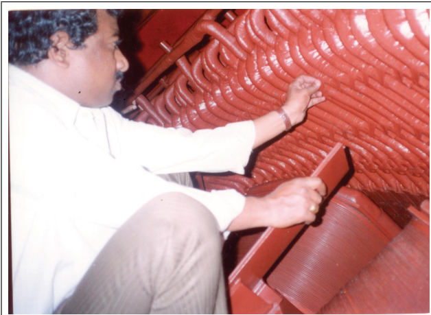
VISUAL GENERATOR INSPECTION OF SABARAGIRI UNIT 4
