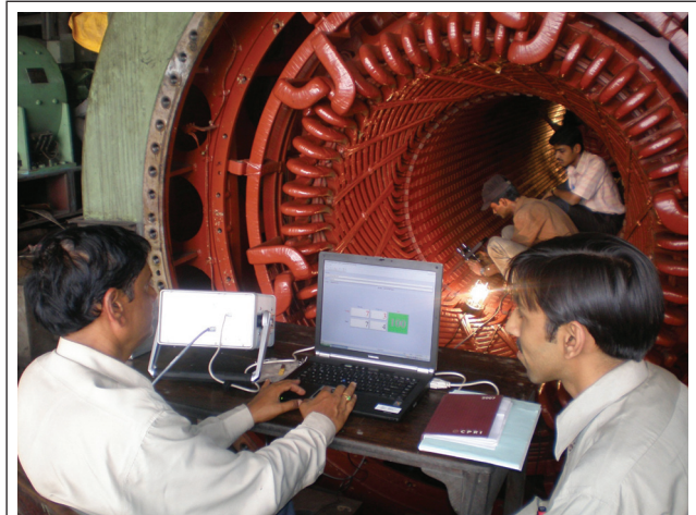
A VIEW OF WEDGE MAPPING TEST IN PROGRESS
