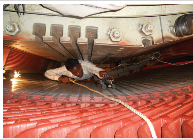
A VIEW OF ELCID TEST ON HYDRO GENERATOR IN PROGRESS
