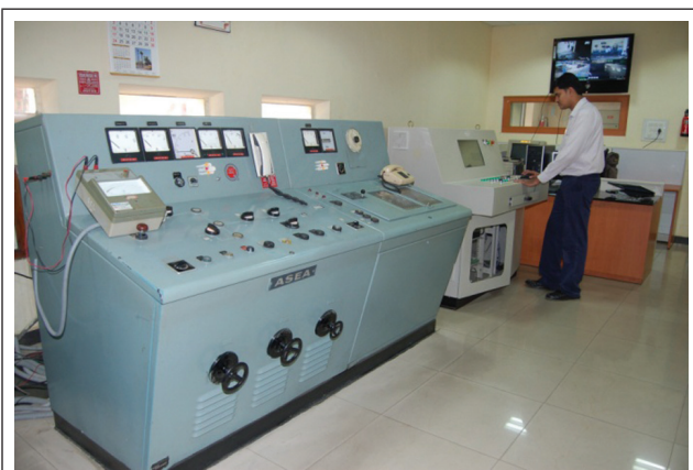
PHOTOGRAPH SHOWS CONTROL ROOM WITH NEW CONTROL DESK AND CCTV SYSTEM
