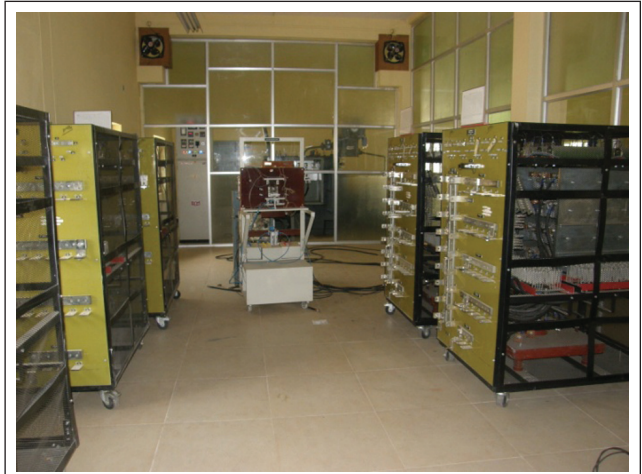
PHOTOGRAPH SHOWING THE NEW 10 kA ON-LINE TEST FACILITY FOR MCB/RCCB TESTING
