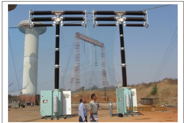
FIG. 31 765 kV - SF 6 GAS CIRCUIT BREAKER
