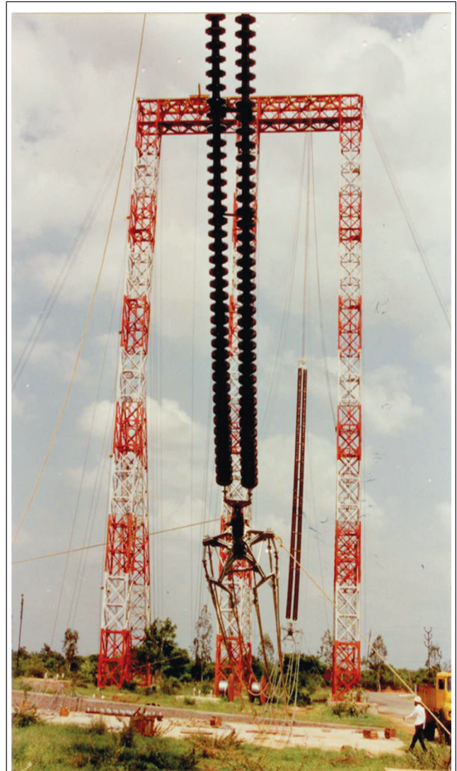
FIG. 7 STRINGING OF 10 SUB-CONDUCTOR BUNDLE IN MOCK UP TEST FACILITY
