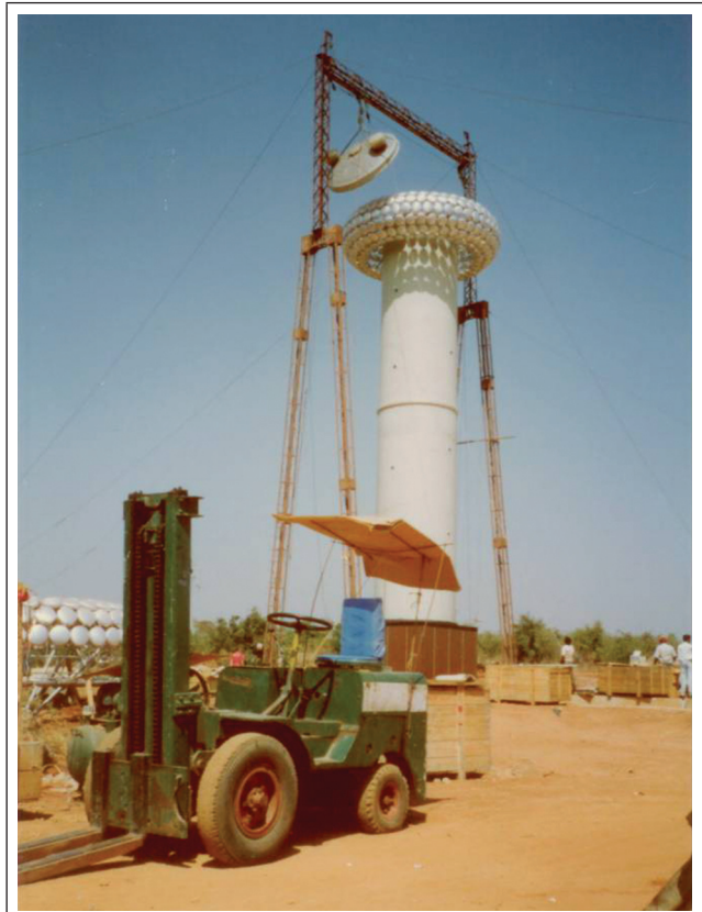
FIG. 1 A VIEW OF OUTDOOR IMPULSE GENERATOR DURING ITS ERECTION
