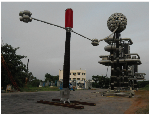
FIG. 26 765 kV CURRENT TRANSFORMER UNDERGOING RIV TEST
