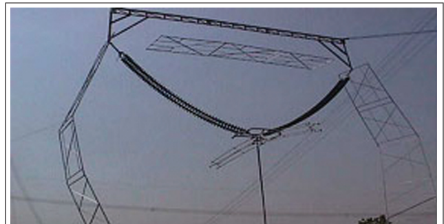
FIG. 4 A VIEW OF 800 kV INSULATOR STRING WITH SIMULATED TOWER
