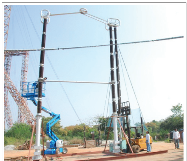
FIG. 33 765 kV - KNEE TYPE DISCONNECTOR
