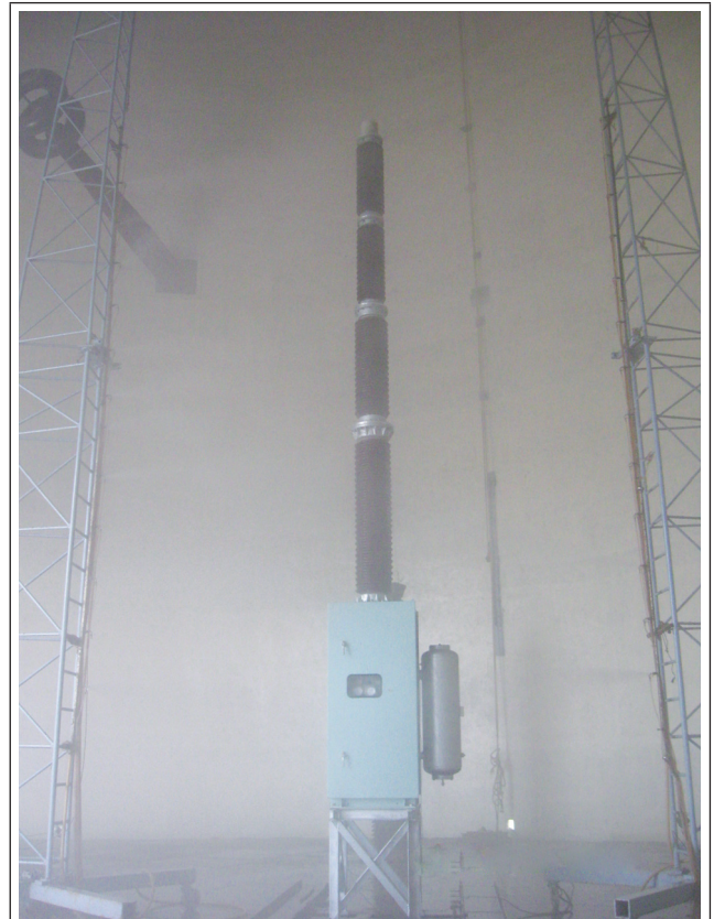
FIG. 36 SUPPORT INSULATOR OF 765 kV GCB UNDERGOING POLLUTION TEST
