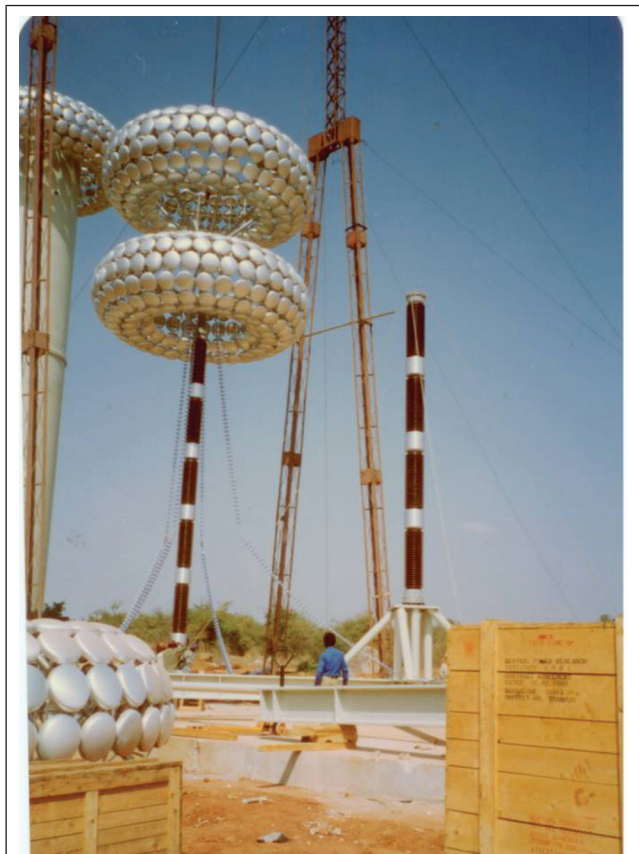
FIG. 2 ERECTION OF 4800 kV DAMPED CAPACITIVE DIVIDER IN PROGRESS
