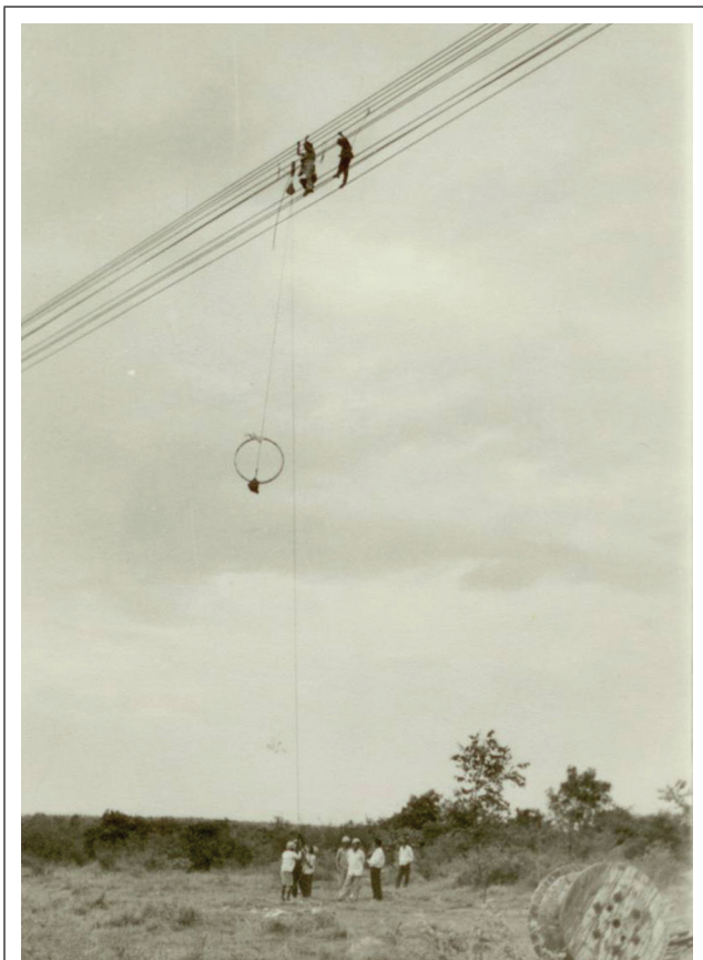
FIG. 19 A VIEW OF CONDUCTOR SPACER BEING ERECTED
