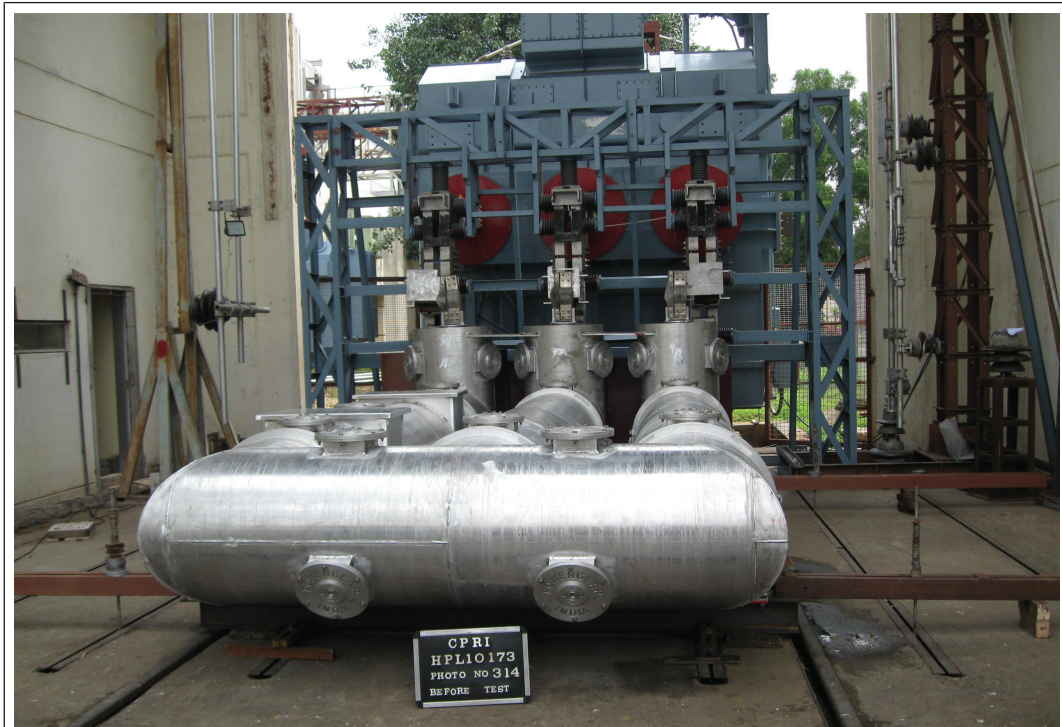
ISOLATED PHASE BUSDUCT TESTED FOR 300 kA FOR 1 SEC
