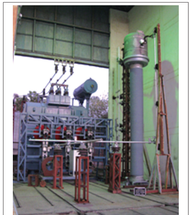
800 kV CT TESTED FOR 50 kA FOR 1 SEC
