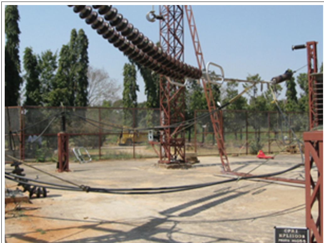
400 kV INSULATOR STRING MOUNTED FOR POWER ARC TEST
