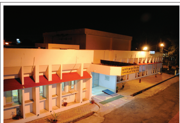
FIG. 36 100 MVA ON-LINE TESTING STN (STATION-2)
