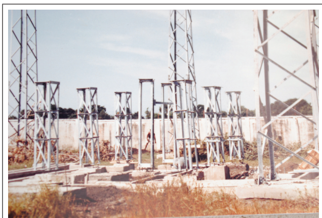
FIG. 28 CONSTRUCTION OF STN-2
