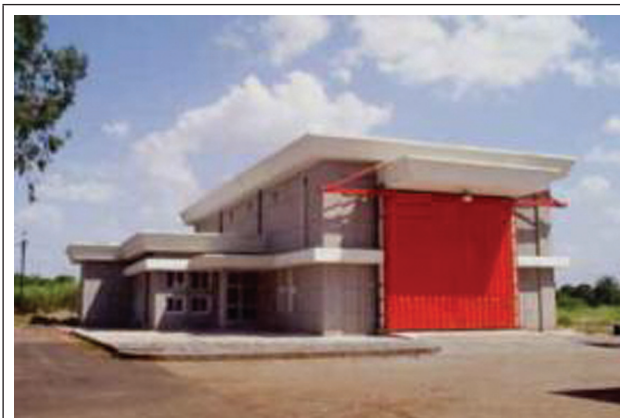
FIG. 10 TEMPERATURE RISE LAB (25 kA)
