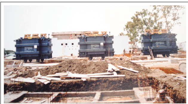
FIG. 4 CONSTRUCTION WORK IN STN-2
