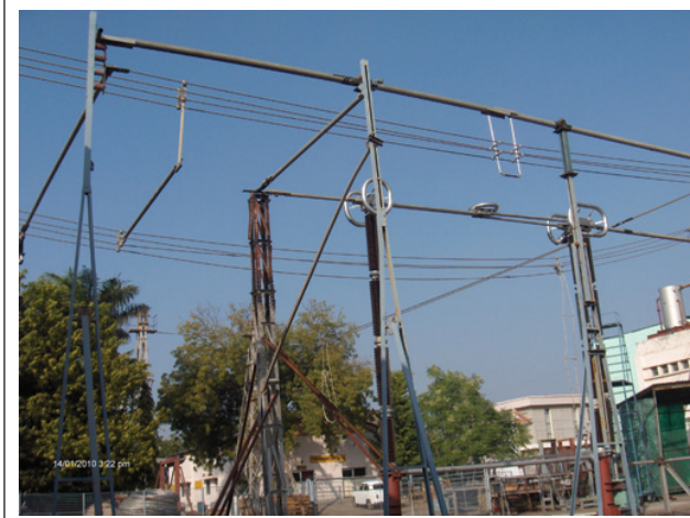
FIG. 16 800 kV, 3150 A KNEE TYPE DISCONNECTOR
