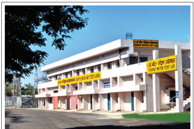
FIG. 38 SUPPLEMENTARY TEST LAB AND ENERGY METER TEST LAB
