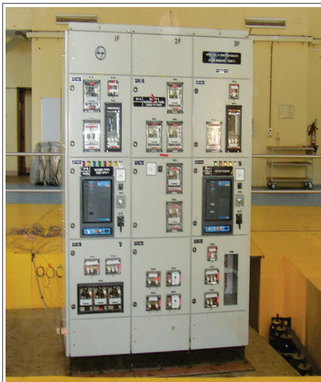
SEISMIC QUALIFICATION TEST
