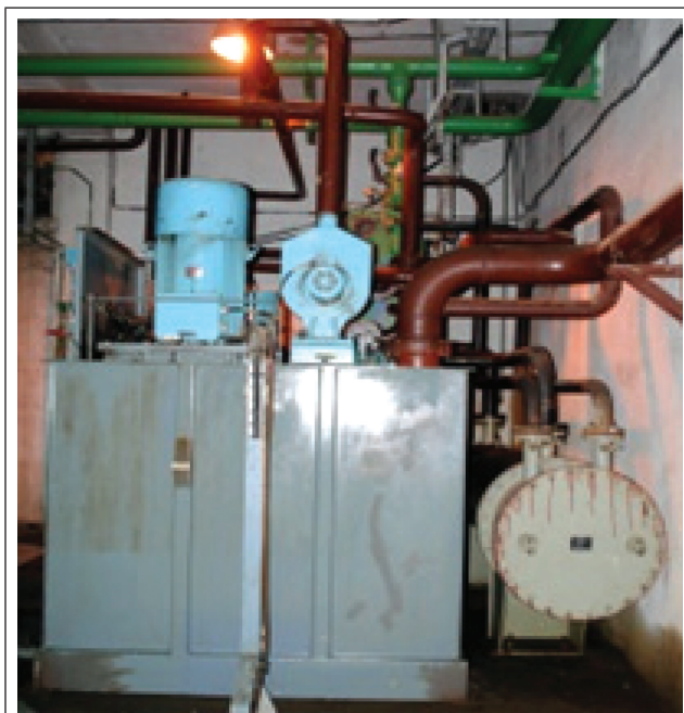
FIG. 9 OIL RESERVOIR AND HEAT EXCHANGER
