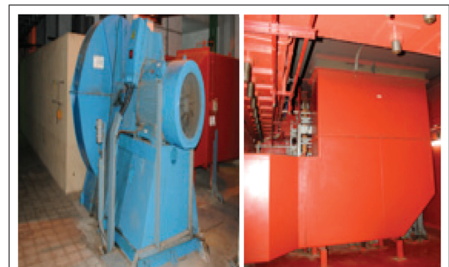
FIG. 7 BLOWER, INLET AND OUTLET DUCT
