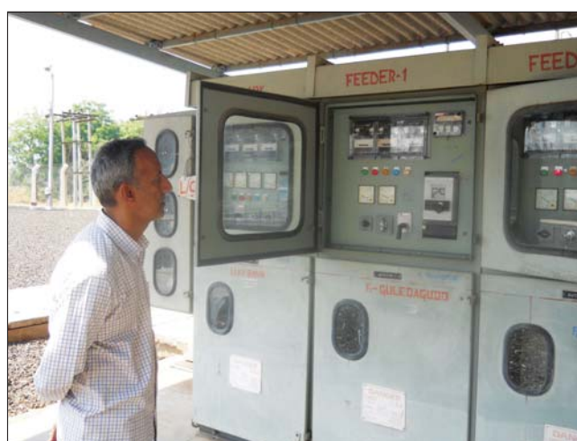
FIG. 2 VERIFICATION OF EXPORT METER
