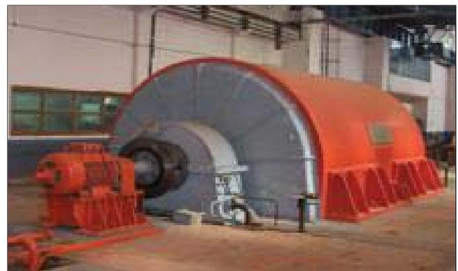
FIG. 14 RE-ASSEMBLED GENERATOR AND OCC THEREAFTER
