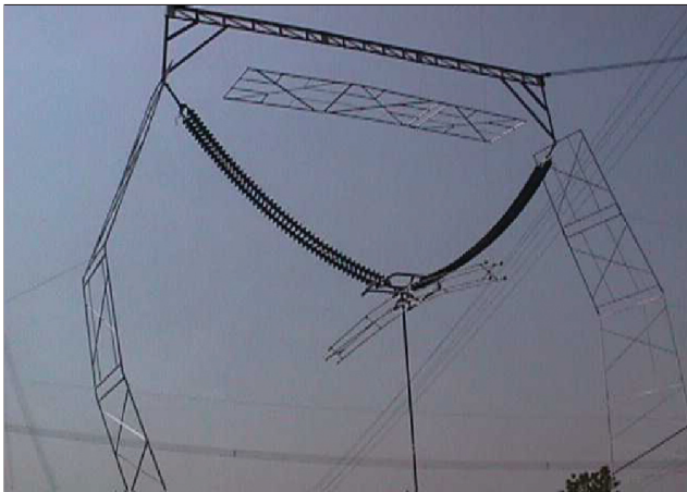
FIG. 8 A VIEW OF 1200 kV INSULATOR STRING WITH SIMULATED TOWER
