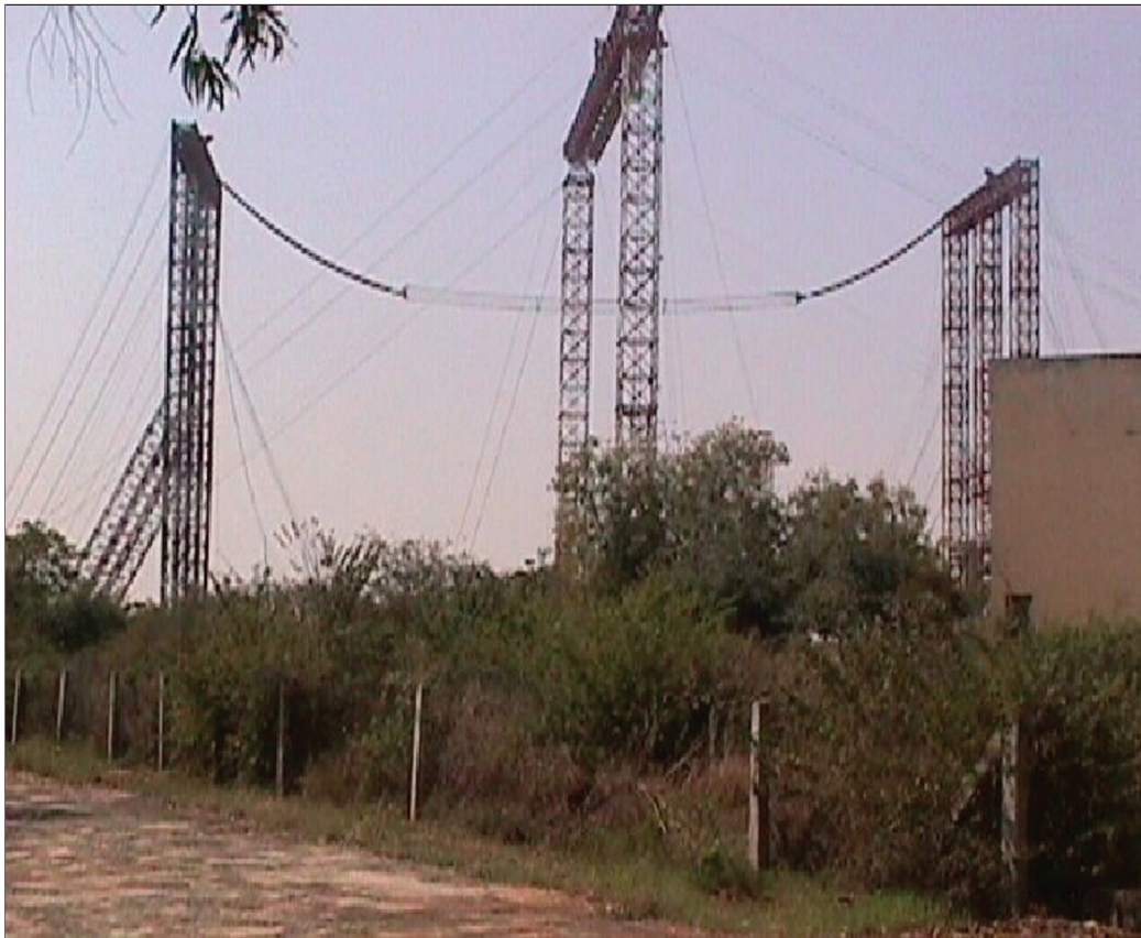
FIG. 9 A VIEW OF MOCK UP TEST FACILITY SHOWING TWO AND THE DIVIDER DEAD END AND CENTRAL PORTAL TOWER
