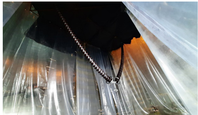
Figure 6. HVDC disc insulators ('V' String).
