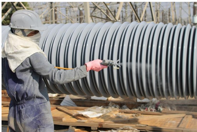
Figure 4. Bushing being coated.
