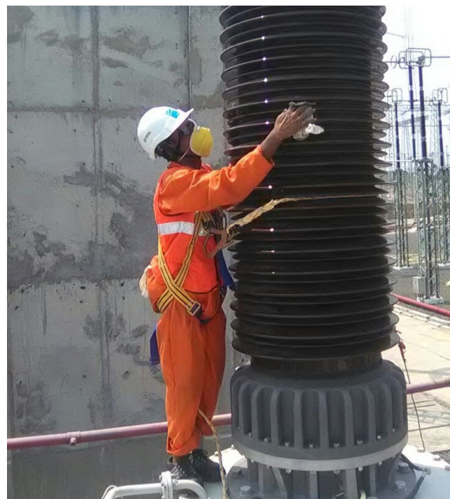
Figure 1. In-situ cleaning of the bushing.
