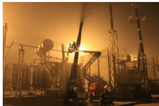
Figure 2. Coating of the bushings.
