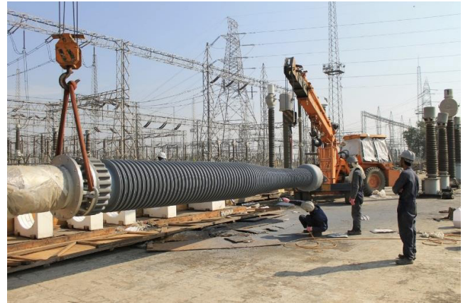
Figure 5. Handling coated bushing.
